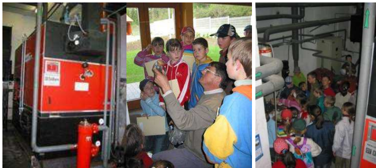
The new biomass heating boiler
